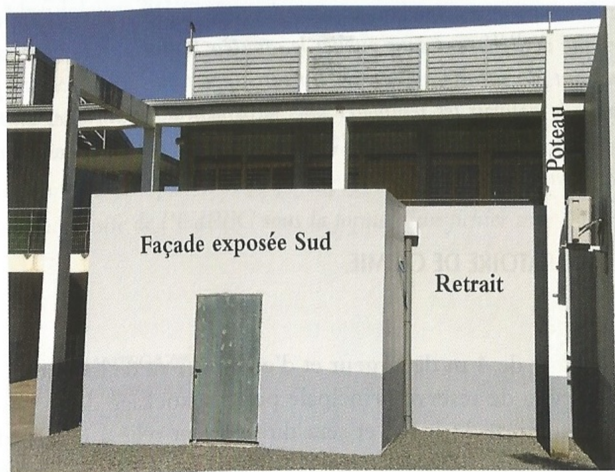
Figure 2 - La façade principale.
